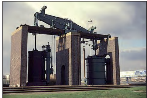
1817 beam and blowing engine
