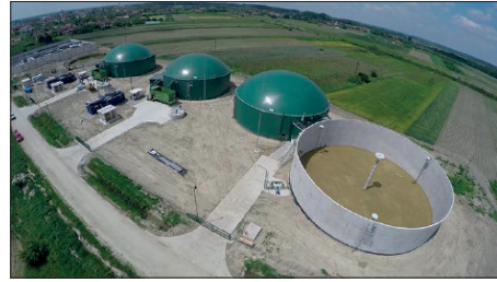
Fig. 6. Three biogas installations in Bač with digestate reservoir
