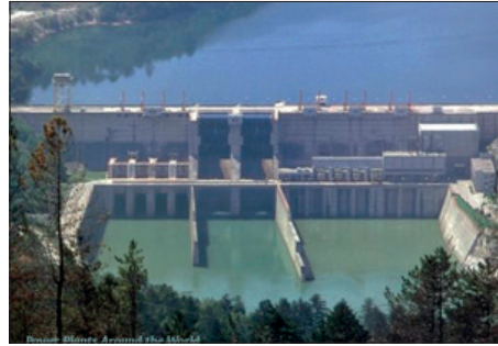
Fig. 2. Hydropower plant Višegrad on Drina, 1989
