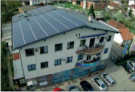
Fig. 3. PV solar power plant BLC 1 of 20 kWp, (2012) and BLC2 of 10 kWp, (2014) Banja Luka
