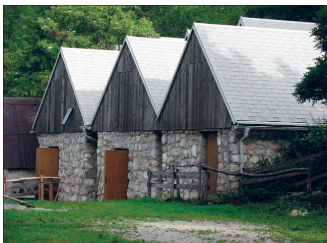
Figure 2: Stables after renovation; the Kuhinja alp. Author: Špela Ledinek Lozej, 2011.
