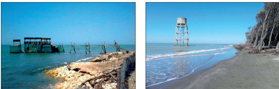
Fig. 2 — Semani beach, a caffe-bar improvised over concrete basements of an old borehole, and a water tower, both were well far from sea one upon a time.
