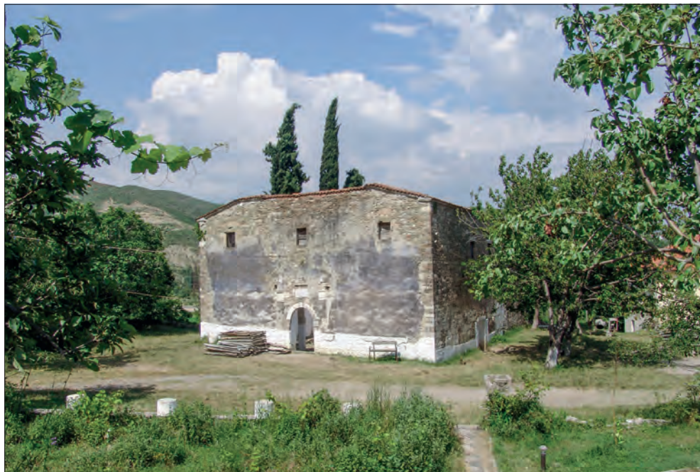
West — South view of the church before restoration
