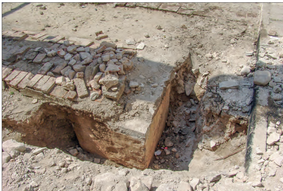
View of the foundation of the column during survey
