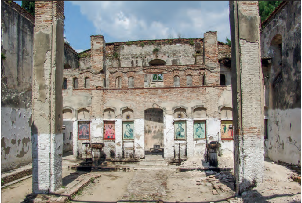
Interior view of the church before restoration
