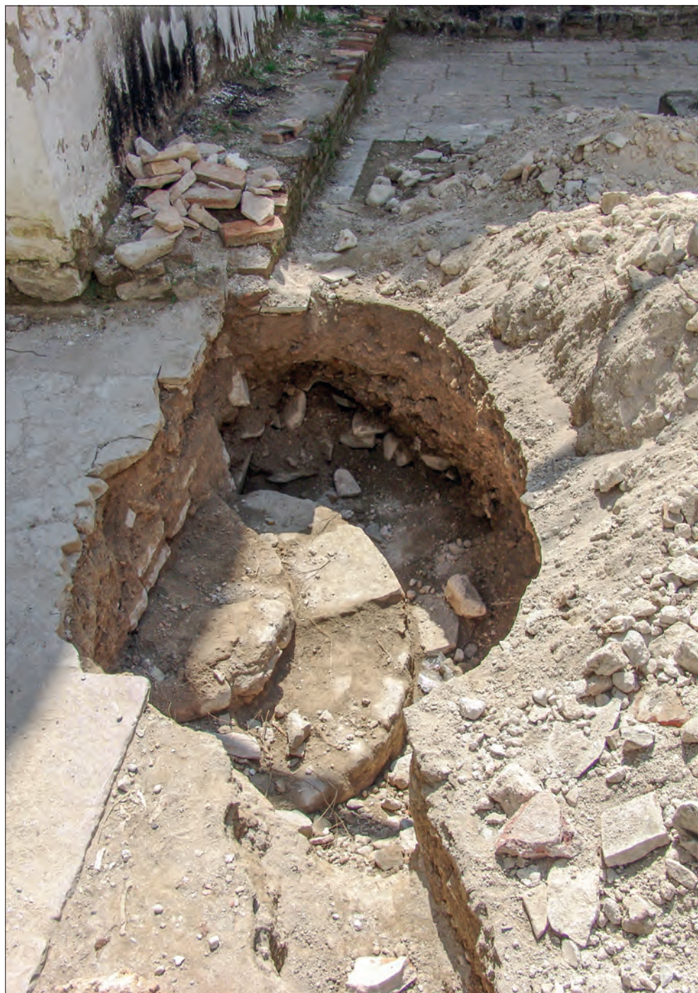
View of the old stairs during survey
